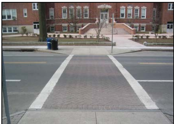
Standard Brick Paver Crosswalk At a School in Greenwich, CT
