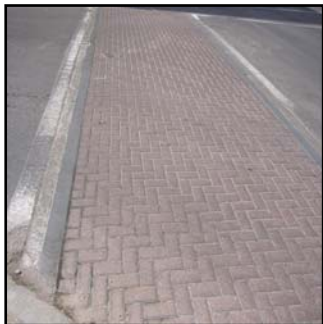
Brick Paver Crosswalk
