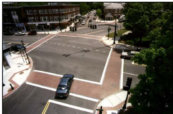
Standard Imprinted Crosswalk Layout
