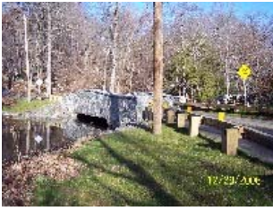
North Porchuck Road Bridge
