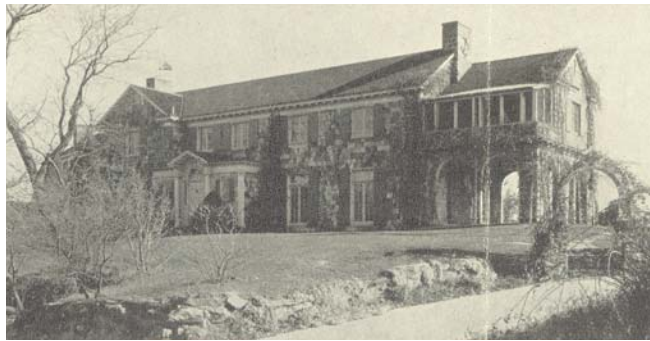
The Anchorage, located in Byram, was constructed in 1925. Photo courtesy of Anthony Chiapetta.
