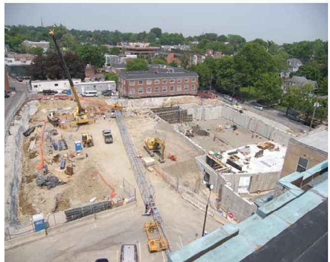
Construction Site, June 1, 2007
