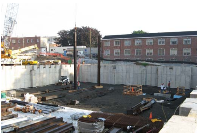
Steel Erection, June 5, 2007
